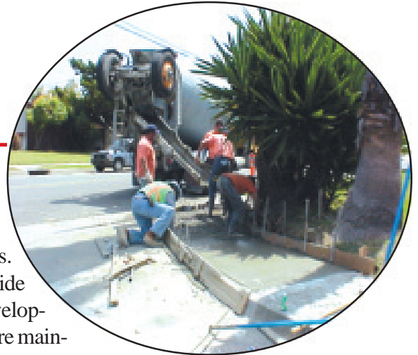
Above: A public works maintenance crew installs a handicap ramp.
