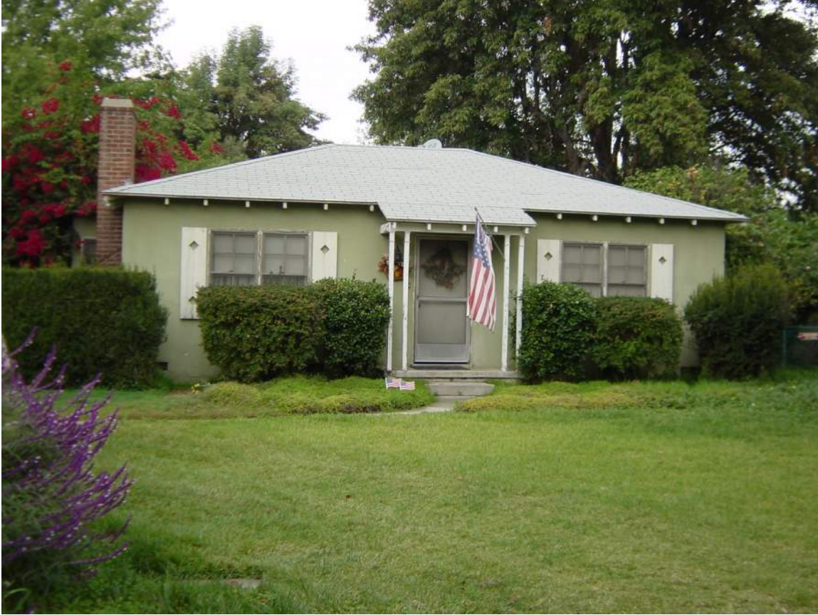
Figure 22. 921 S. Sunkist Avenue
