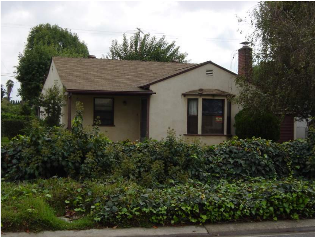
Figure 21. 1010 S. Sunkist Avenue
