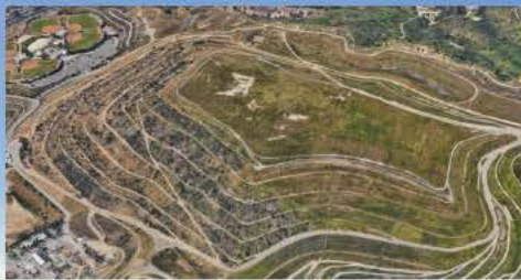
The closed BKK Class III Landfill on Azusa Avenue...
