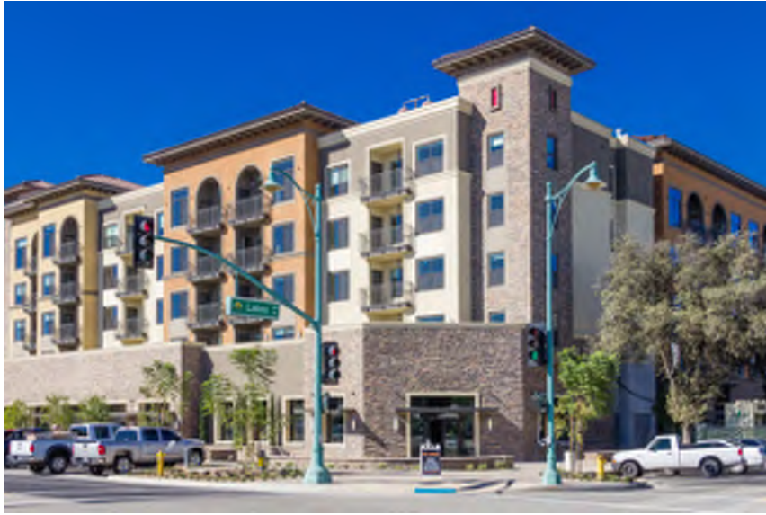
The new 5-story mixed-use development adds 450 units and 20,000 square feet of retail space to the Downtown area.
