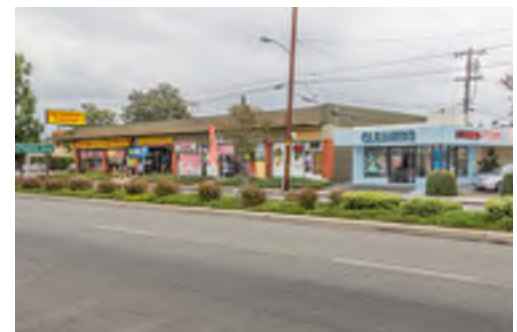
Retail on North Azusa Avenue
