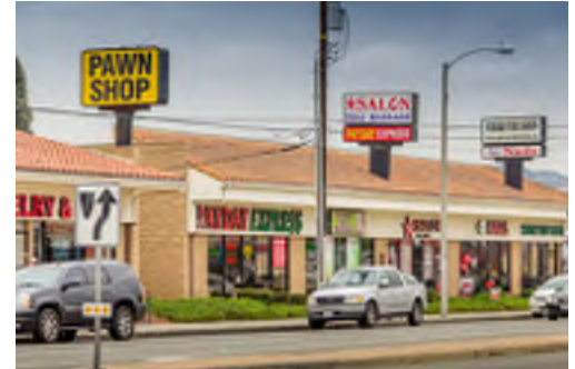
Retail on North Azusa Avenue
