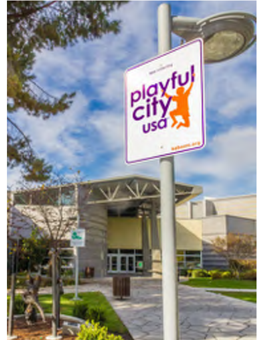
Cameron Park Community Center
