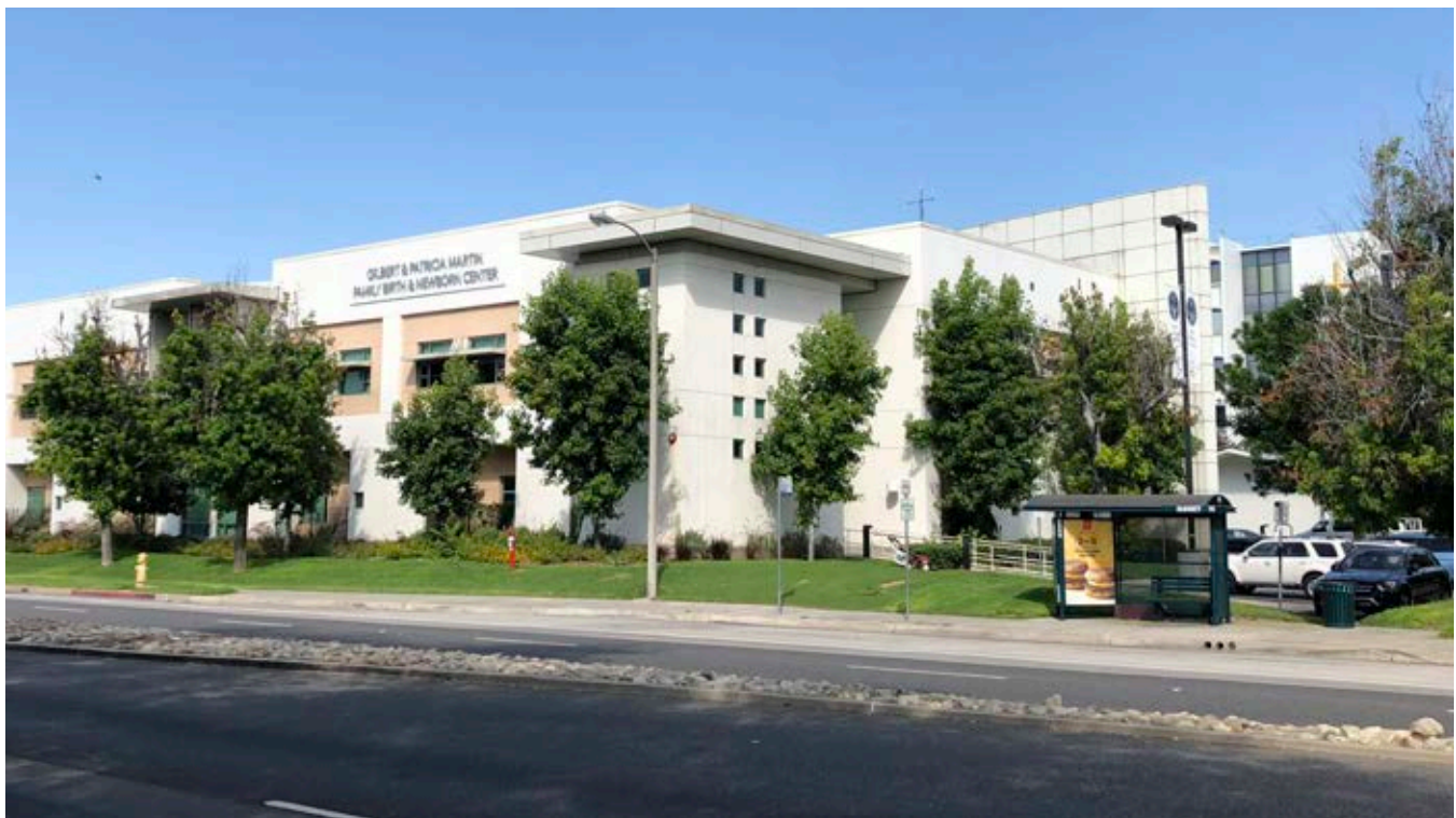
Existing Queen of the Valley Hospital buildings along S. Sunset Avenue.
