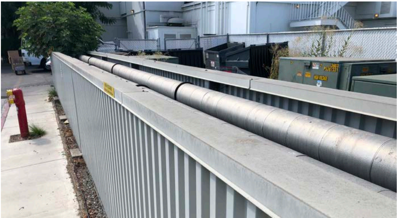
Waste Disposal Bins and Electric Boxes Screened Behind a Metal Wall
