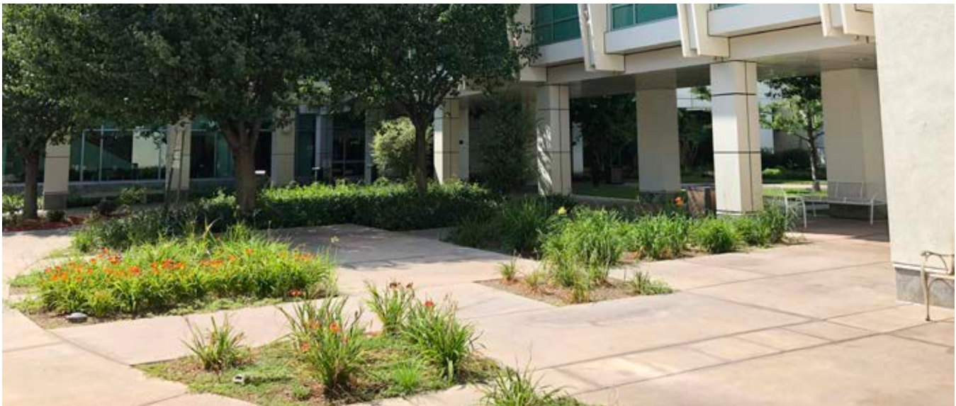
Stained concrete with landscape pockets and metal benches
