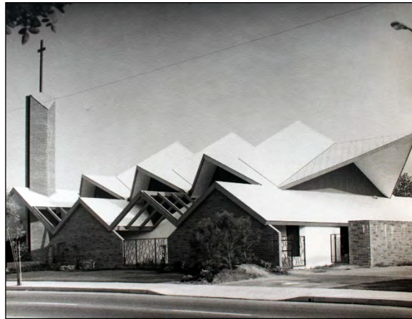
Figure 33. West Covina Christian Church, no date (Source: West Covina Historical Society)
