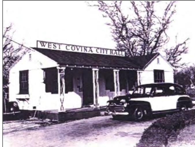
Figure 2. In the 1940s, this house (demolished) in the Sunkist Village development also functioned as City Hall. (Source: West Covina Historical Society)
