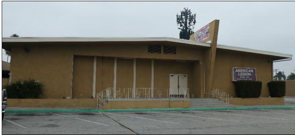
Figure 36: American Legion Post 790, originally constructed as the Citrus Municipal Court in 1956, 2019 (Source: GPA)
