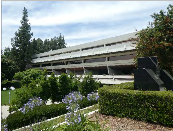
Figure 51. West Covina City Hall, 2019 (Source: GPA)
