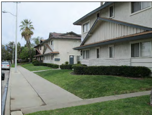
Figure 22: A typical multi-family apartment in West Covina, relatively low-scale and stylistically similar to nearby single-family homes, 2019 (Source: GPA)
