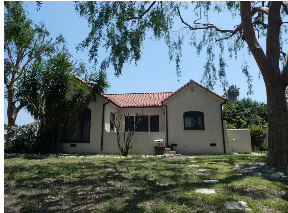
P5b Description/Date of Photo Northwest elevation, view facing southeast/2019
