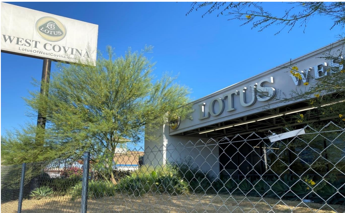
View of existing Lotus dealership building located at the southwest corner of the project site.
