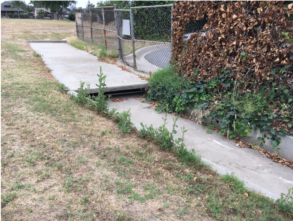
Photograph 7: View of the concrete-lined storm drain on the project site.
