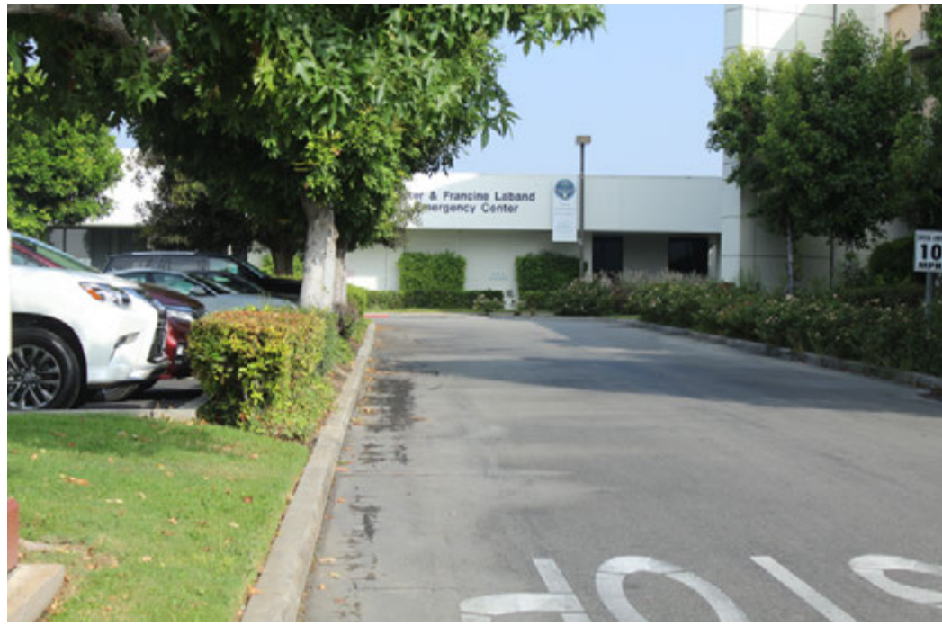
View 7 - Looking west into southern entrance off of Sunset Ave.
