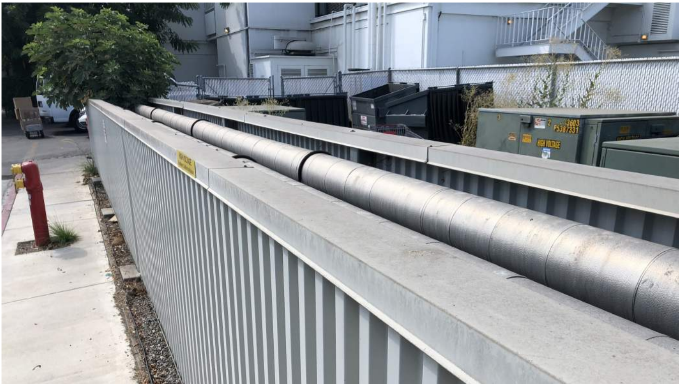
Waste Disposal Bins and Electric Boxes Screened Behind a Metal Wall
