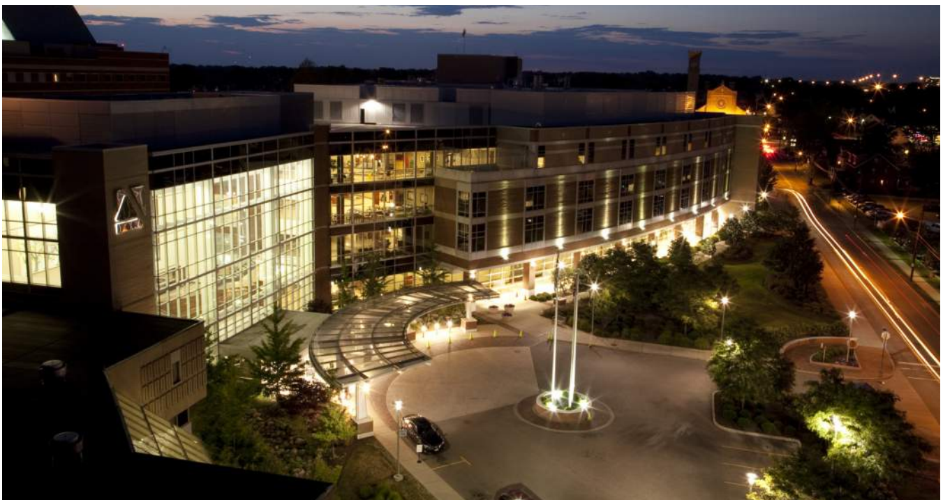
Example of building lighting using a variety of methods
