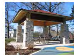
COVERED SHADE STRUCTURE
