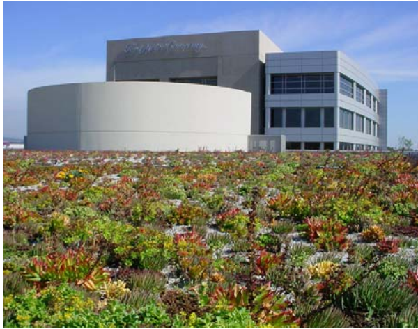
Figure IV-2. Green Roof of Premier Automotive Group in Irvine, CA. Source: Roofscapes Inc., 2004
