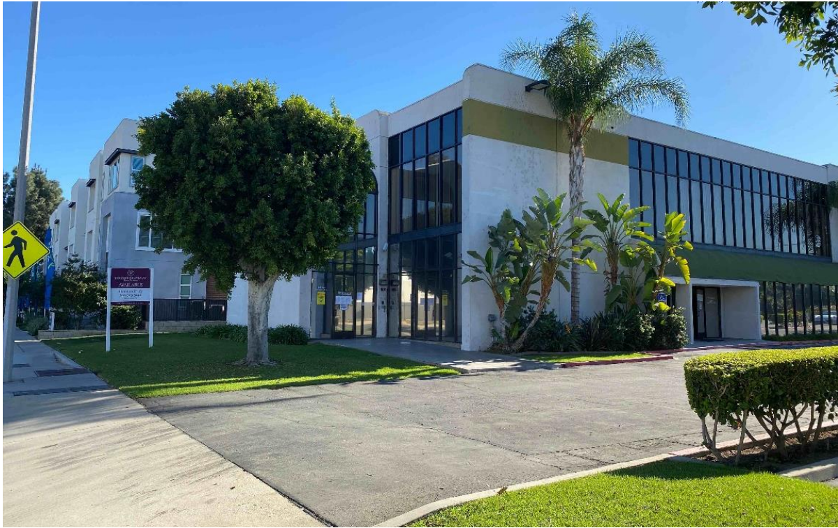
Photograph 9a. Existing office building at 1600 West Cameron Avenue
