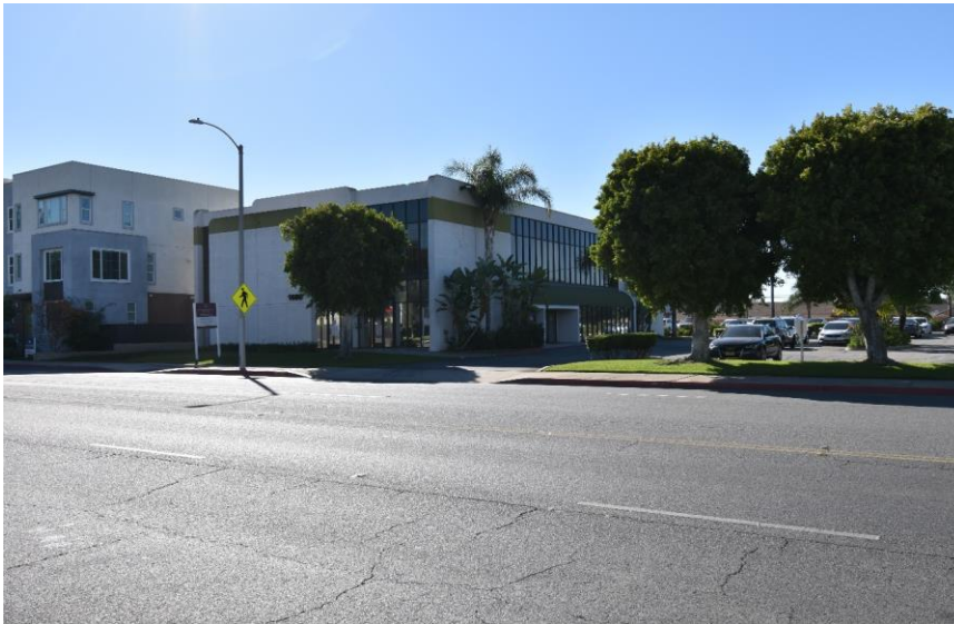
View of building from West Cameron Avenue, December 2020.
