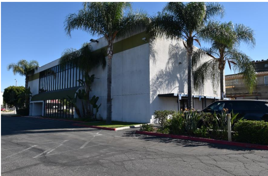
South and West Elevations, December 2020
