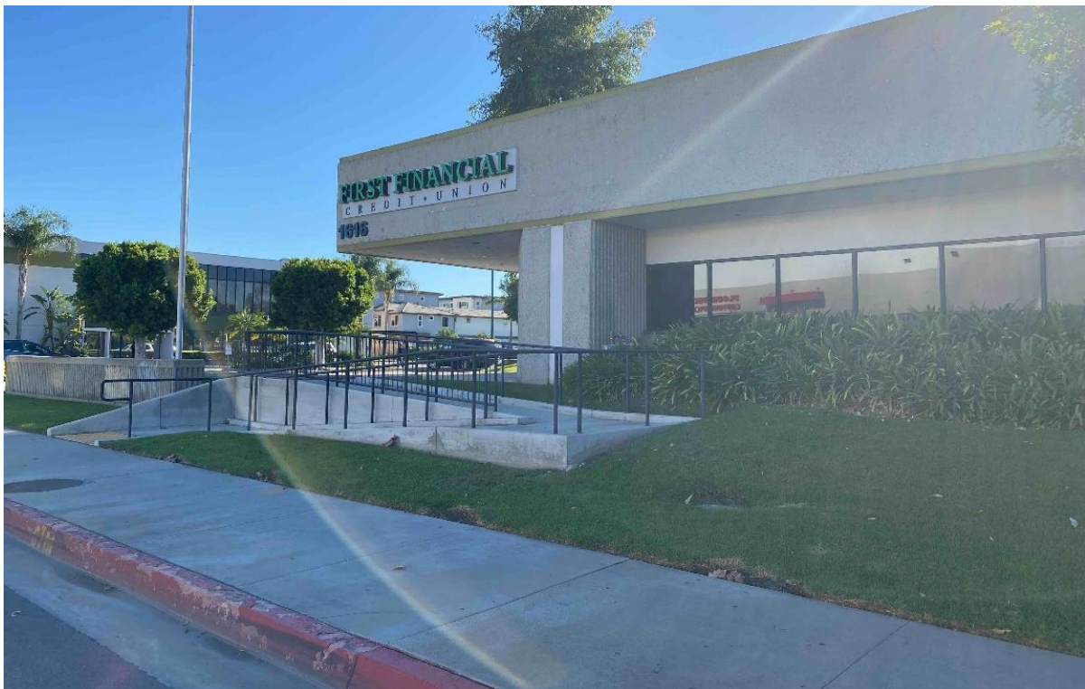
Photograph 9b. Existing office/commercial building at 1616 West Cameron Avenue
