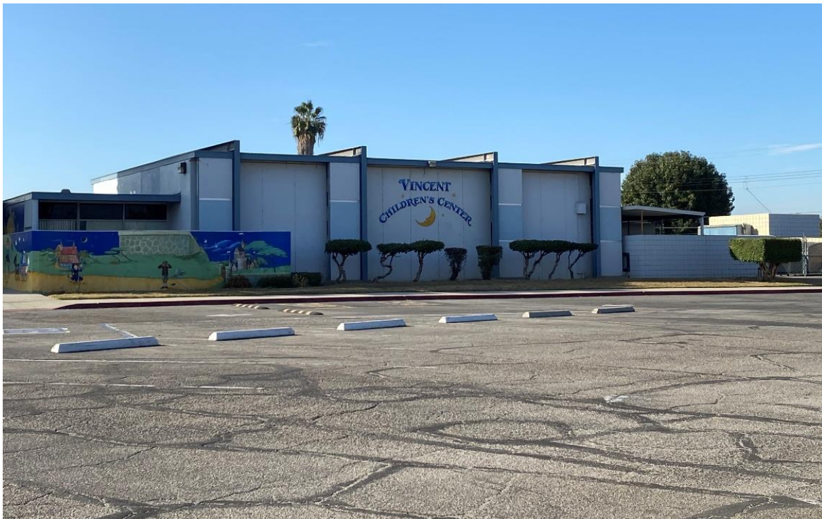
Parking lot and Vincent Children's Center in the northern portion of the site.
