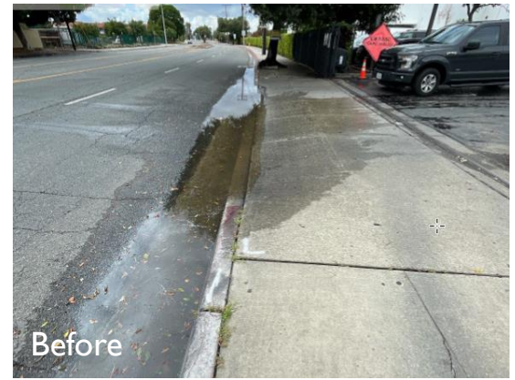
2009 W. San Bernardino Rd | Driveway Approach, Sidewalk & Curb-Gutter Repair
