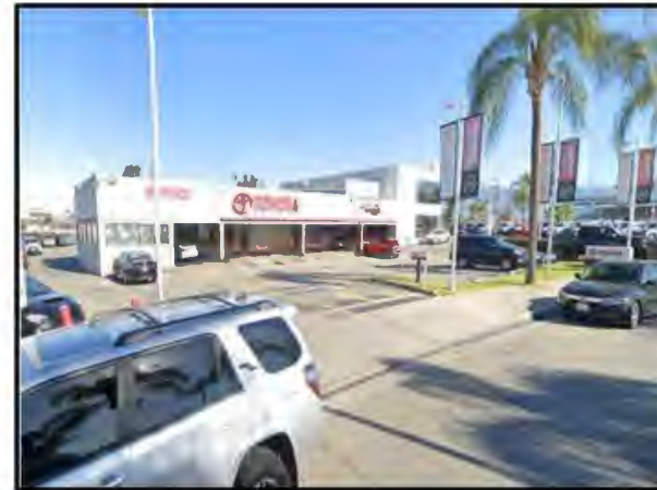
PHOTO 2: View looking at the eastern portion of the project site along East Garvey Avenue.
