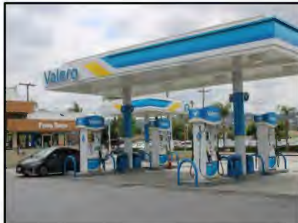
PHOTO 3: View looking at the southern portion of the project site along East Garvey Avenue.
