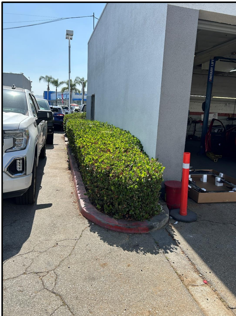
Figure 4.3-3 HEDGE LANDSCAPE BED ON NORTH SIDE REPAIR SHOP; VIEW TO THE EAST
