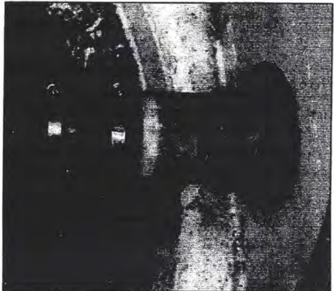
FIGURE 5-1. Boots on piping transitions and through sump walls must be leak-tight when piping secondary containment integrity testing is performed.
